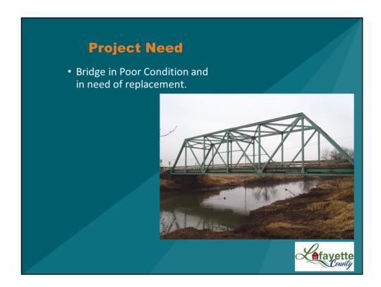
The existing bridge constructed in 1938 is in poor condition. It has a sufficiency rating of 42.1. Sufficiency rating is a measure of the condition of a bridge on a scale of 0-100 which considers many factors including the condition of the bridge itself as well as other functional information including roadway width, clearances, etc.
